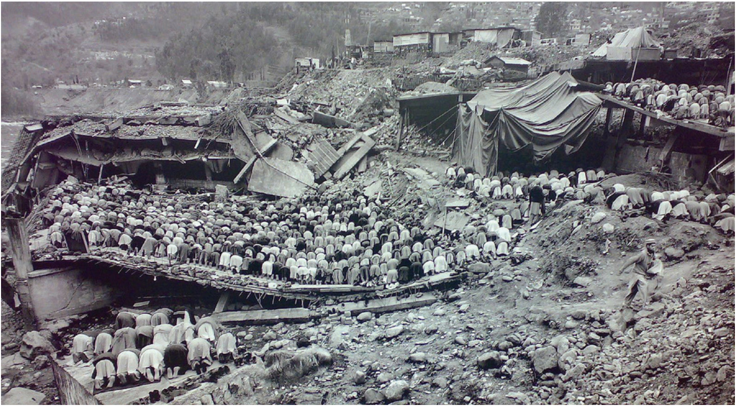
People attend Friday prayers on what remains of a mosque following the 2005 earthquake
